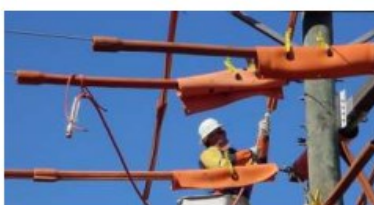
Figure 14 Blankets wrapped and pinned
