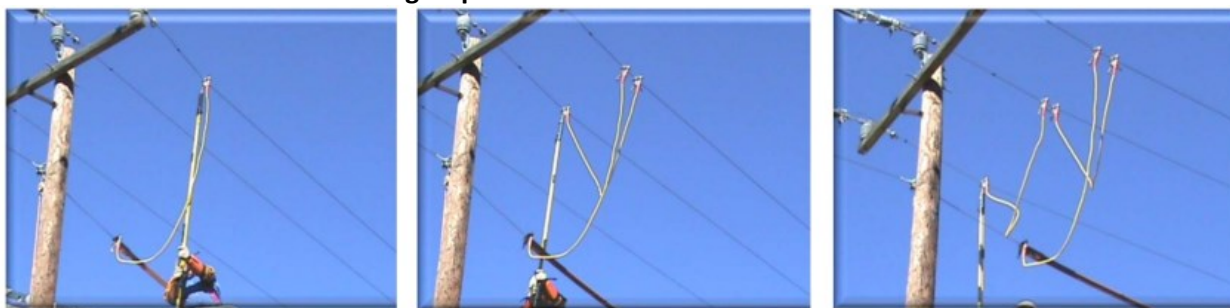
Figure 27 Grounding in steps
