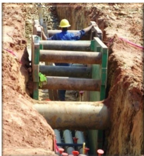
Figure 41 Shoring Protective System
