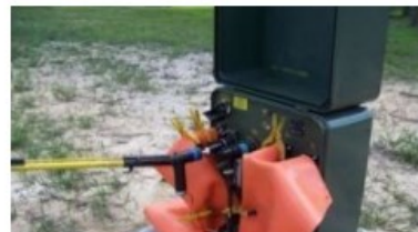
Figure 15 Blankets used in underground work
