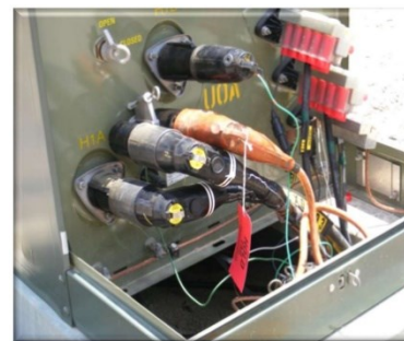
Figure 35 Grounding URD Equipment
