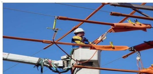
Jumper end secured with T-Handle
