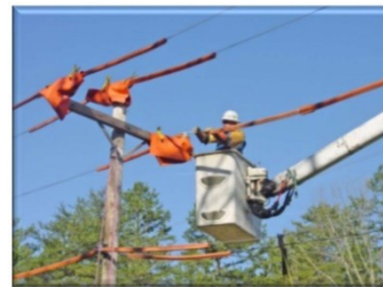
Figure 10 Installation of Cover Up
