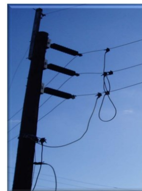
Figure 29 Chain Grounding (Daisy Chain)
