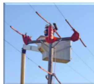
Figure 12 Blanket wrapped Conductor & Insulator
