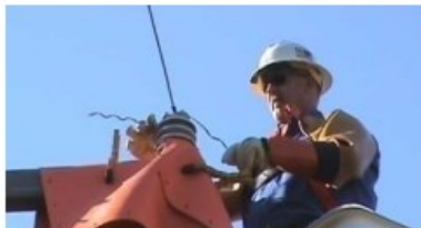
Figure 13 Split blanket used to cover Cross arm & bottom of insulator
